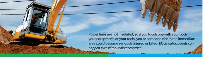
Whether you operate heavy equipment or use ladders and handheld tools on the jobsite, it's critical that you keep a safe distance from all power lines and electrical equipment while you work—at least 10 feet, and possibly more depending on voltage.
